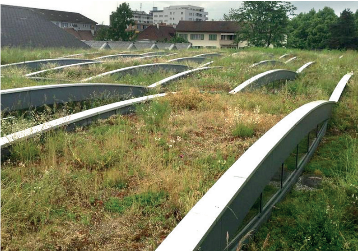
Undulating Green roof that has a variety of soil depths.
