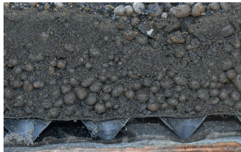
Green roof substrate cross section
